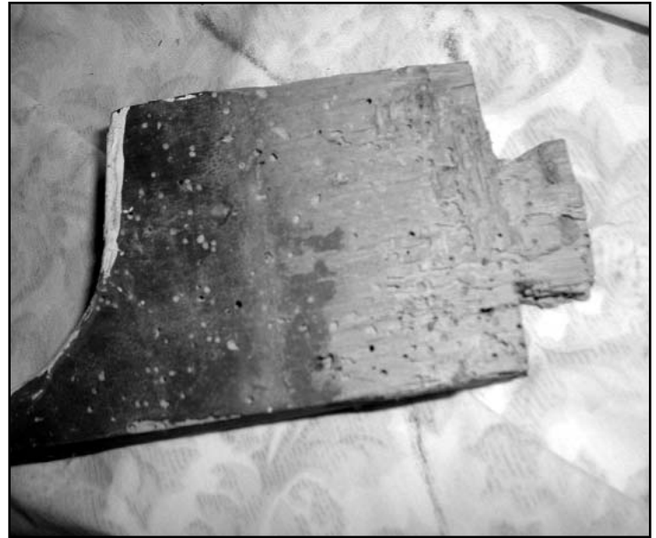
Figure 2. Wood borer damage.
