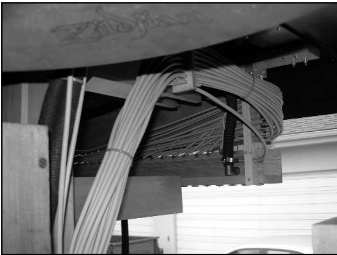
Figure 26. Backside of installed chest, showing main vacuum supply and key action tubes (dressed towards the back).
