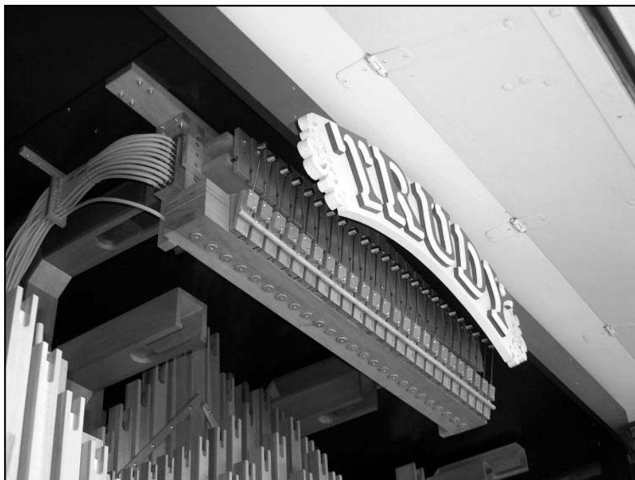
Figure 24. Final installation of bell chest.
