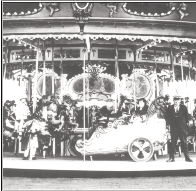
Figure 1. PTC#30 at Luna Park, Melbourne photographed in 1923 showing the organ façade in the center of the carousel. Note the addition of the figurehead and the missing top sections.
