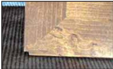
Figure 4. Notched corners in the bottom board to accommodate the hinges.
