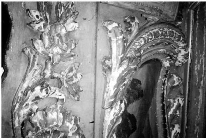
Figure 2. A close-up of one end of the lower facade panel showing the distressed original paint. All carvings looked like this.
