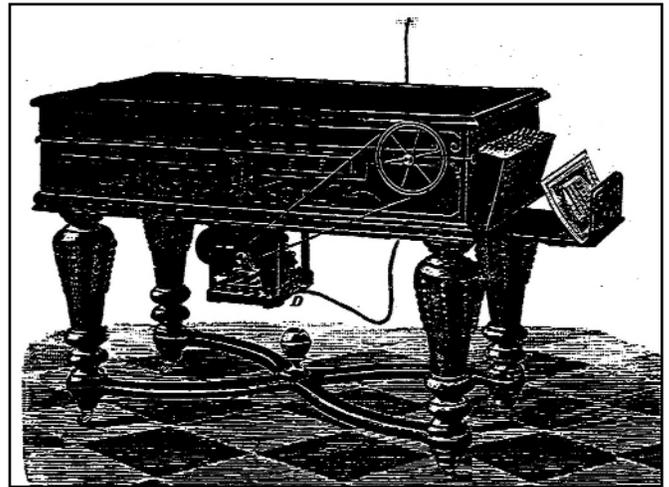
Figure 6. Piano Melodico, 30 notes, with electric motor drive (from catalogue “Holzweissig,” 1898).
