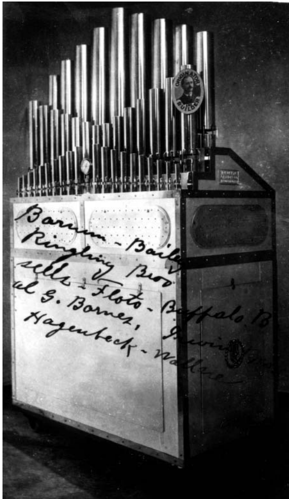
Figure 3. This is the standard 43-whistle air calliope that evolved after a few years. The keyboard and siren whistle were located behind the whistles. Ori inked the names of some of his satisfied customers on the print.
